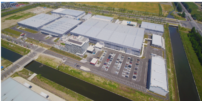
The new site in Nantong (China) has proved its worth and the anticipated efficiency gains have been realized.
